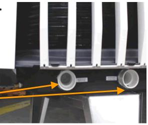
Water inlet and outlet pipes
